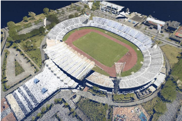
Dense LiDAR points in RGB colour over Stadium Sultan Haji Hassanal Bolkiah in Brunei & Muara District, Brunei Darussalam. The colour was imported from the aerial imagery of the stadium. Image courtesy of Soartech Systems.
